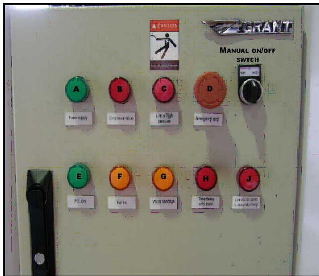
Control Panel on B400 Bin with Manual On/Off switch fitted
